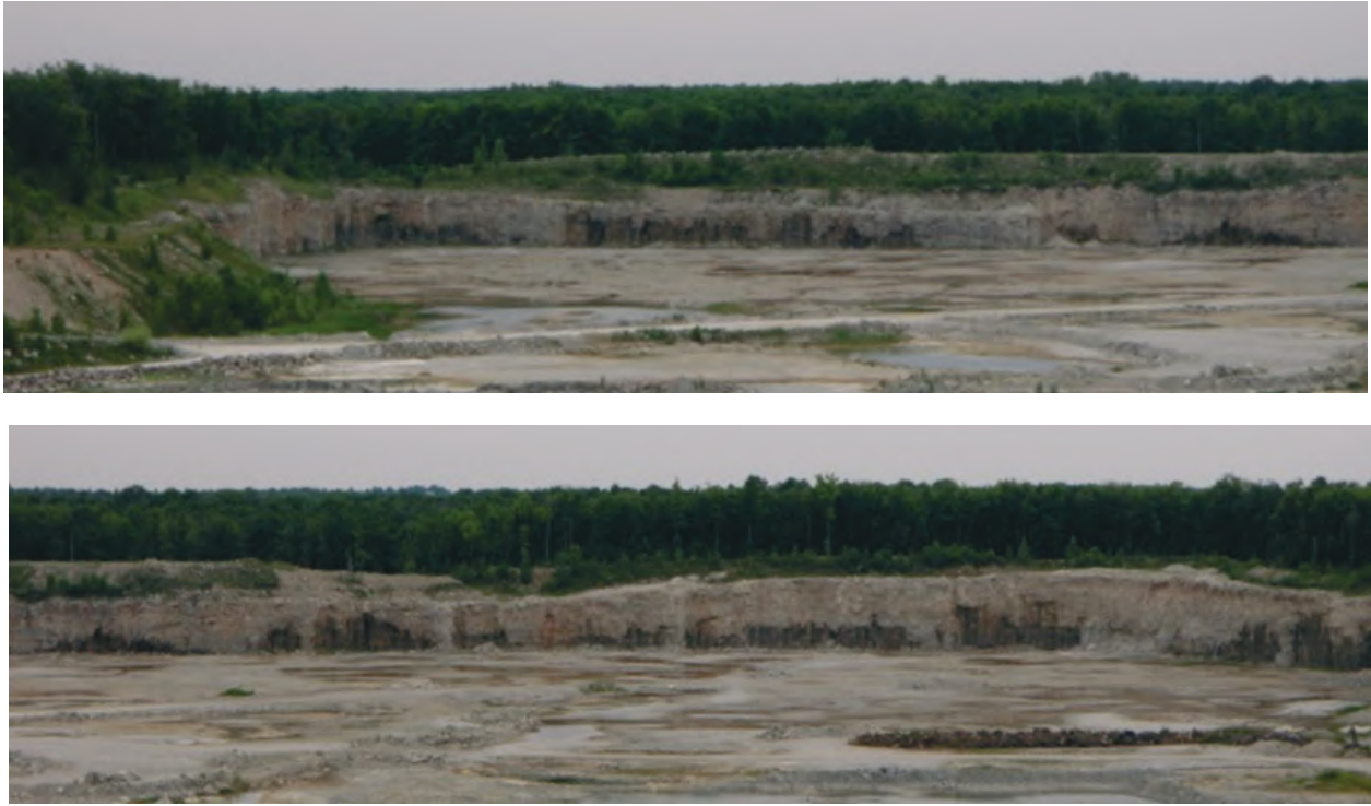
Figure 3. View westwards across Milton North Quarry, showing the southern part (top) and the northern part (bottom) of the quarry face. The widespread dark-coloured areas show that distributed nature of discharge from the quarry face.
