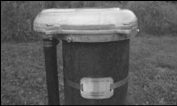
Above: New style vermin proof cap for dug or bored wells. Below: Vermin proof cap for drilled wells.
