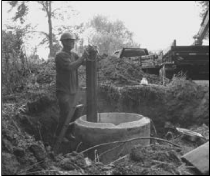
Well upgrade in progress.
