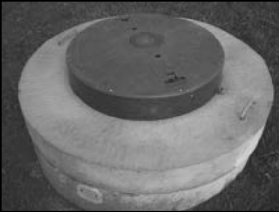
Above: New style vermin proof cap for dug or bored wells. Below: Vermin proof cap for drilled wells.
