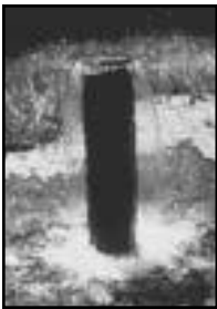
Flowing well that is not controlled.
